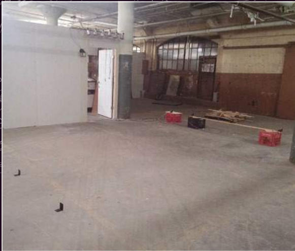
Above left Significantly less scary with the lights on, nevertheless you can see the motion sensors mounted on crates that make it work
