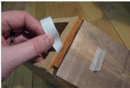
Fig 6 Slide the camera cable between the roof hinge and the back wall of the box
