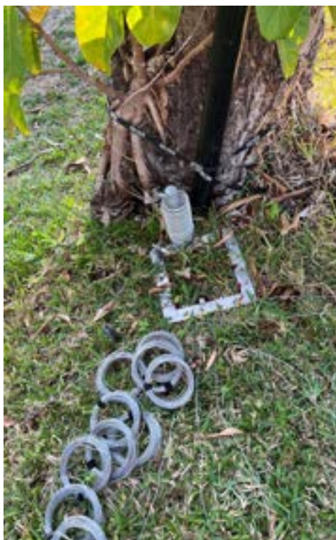
160m vertical matching unit and radials
